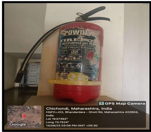
Fire Safety Cilendar
