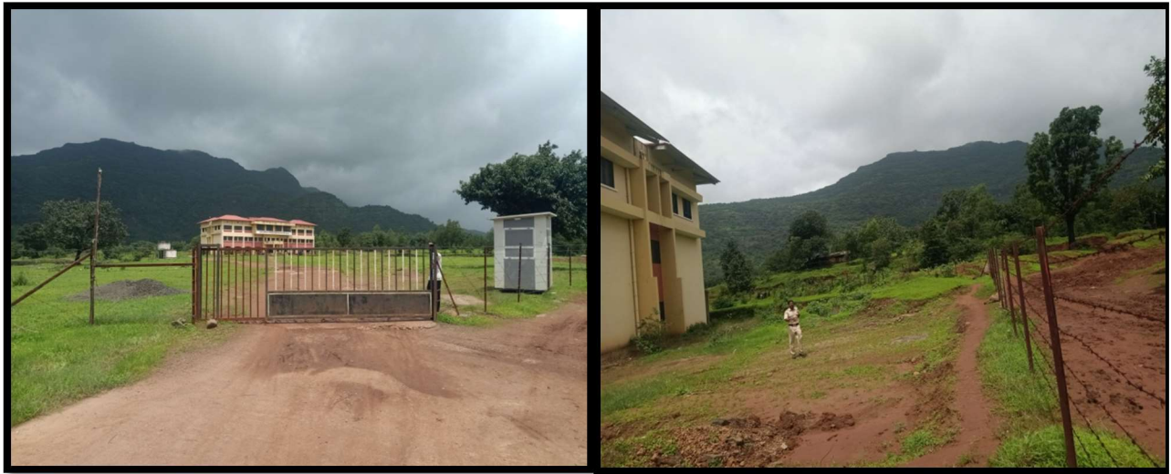
College Gate &Compound
